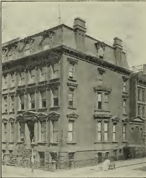
B'nai B'rith Building, New York. (From a photograph.)
