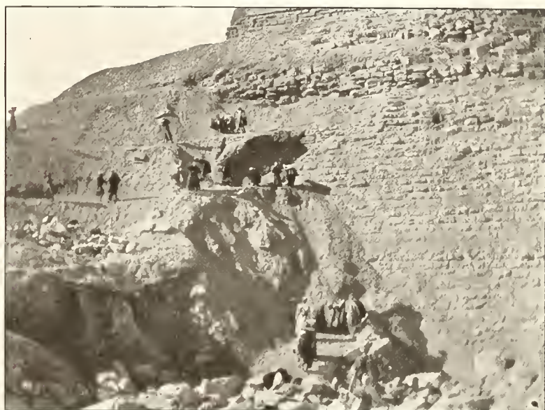
3 CLEARING PYRAMID, EAST FACE.
